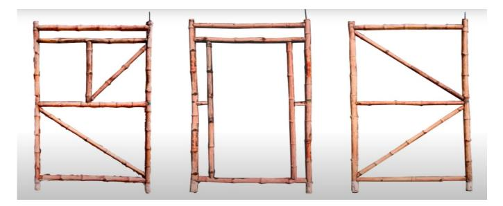
They are inserted directly into stem walls. Holes are made in the place where bamboos are going to fit in. The perimeter of the hole is then filled with lime sand and aggregate mixture in the ratio of 1:3:6. In this way, the walls are going to be fitted very well in the stem wall. The walls panel is then fitted with some thatch material and later on plaster is done using lime mortar or mud mortar.
